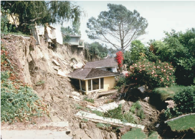
(A) This photograph shows the upper part of a landslide in California, where homes were displaced along the curved rupture surface of the slump block. (Courtesy of Geophoto)
