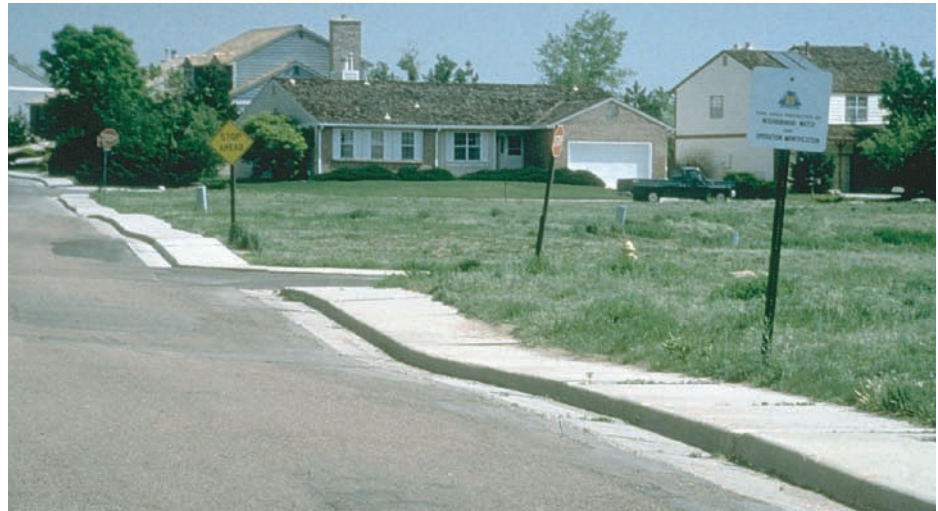
FIGURE 11.16 Subsidence is a major type of mass movement that affects roads and buildings, causing millions of dollars of damage each year. Repeated swelling and contraction of clays have caused this road in Colorado to buckle into waves like a roller coaster. (Courtesy of D. C. Noe, Colorado Geologic Survey)
